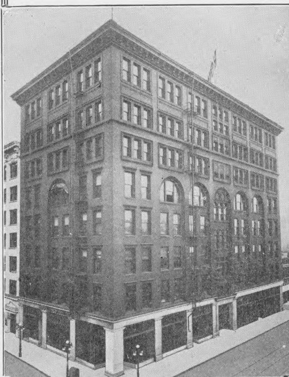
Royal Union Life Building, Cor. 7th and Grand Avenue Des Moines, Iowa
