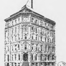
THE BANK'S SECOND BUILDING—1868
