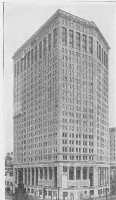
First and Old National Bank, Detroit, Which Has Replaced the Hotel Pontchartrain.
