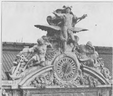
Indiana Limestone Clock Group. Grand Central Terminal, New York City.
