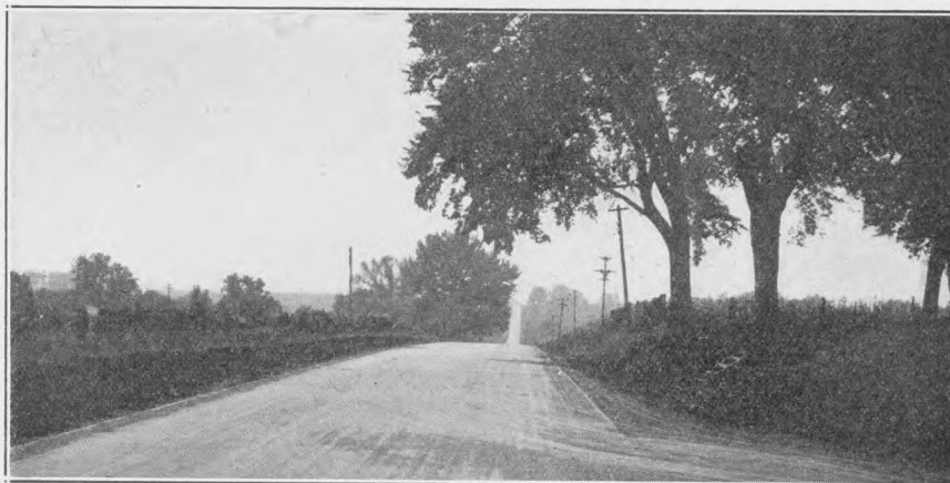
Carlisle Road, Polk County, Iowa. According to figures reported by the Congressional Agricultural Commission, wheat hauling over this type of road, concrete, cost the farmers of the United States, an average of 15 cents per ton while the same hauling cost over an earth road surface costs 30 cents per ton. Tests at Iowa State College show that on this type of road a gallon of gas will give a ton mileage of 31 as compared with 21 ton miles on gravel and 14 ton miles on earth surface. Further, a ton mile on this type of road costs 0.77 cents compared with 1.15 cents on gravel and 1.71 cents on earth, with gasoline costing 24 cents per gallon.
