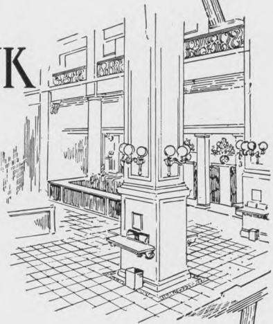
Glimpse of a section of the lobby.
