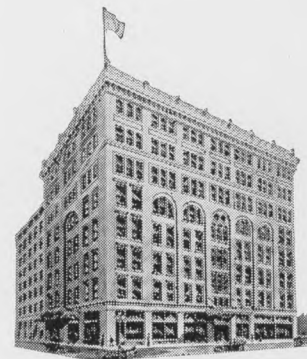
United Bank Building Home of United State Bank
