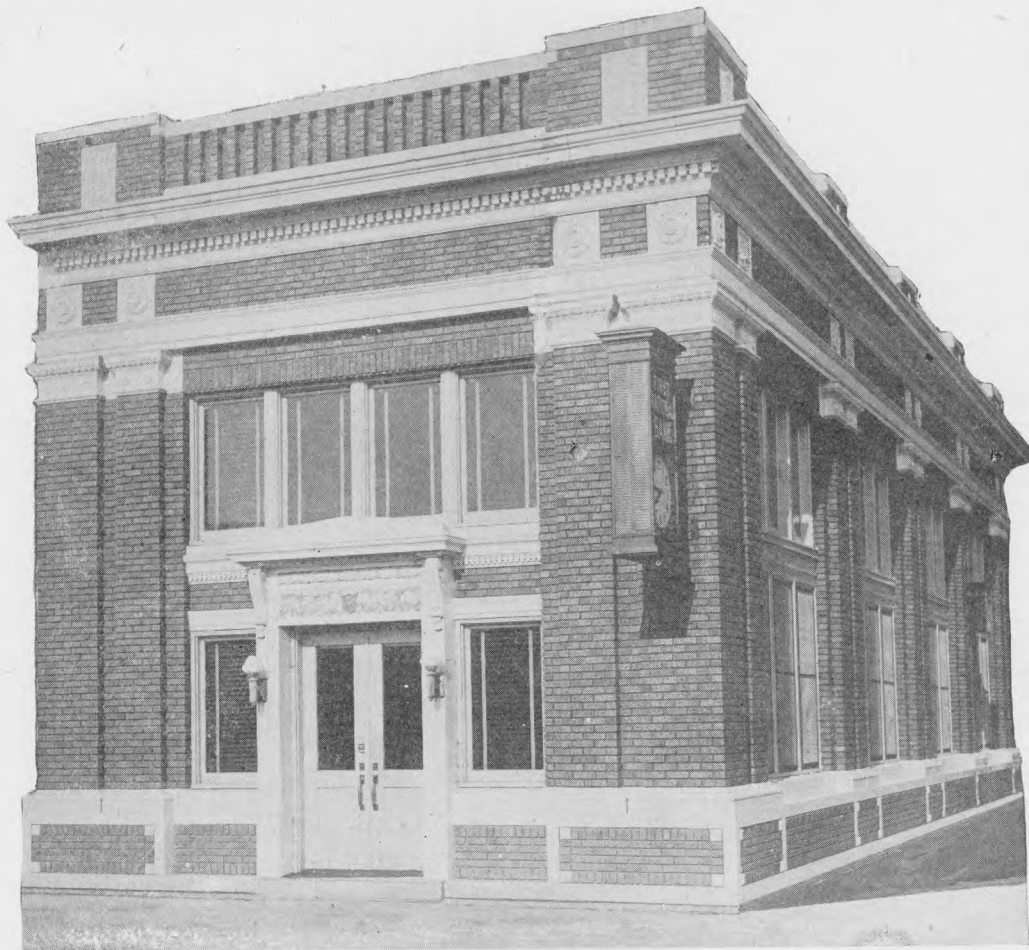
First National Bank, Inwood, Iowa.
