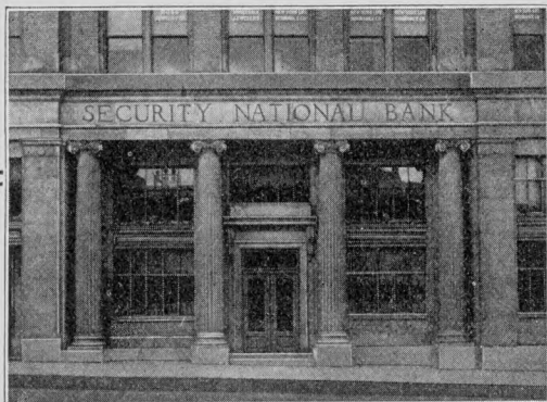
Entrance to The Security National Bank Sioux Falls, S. D.
