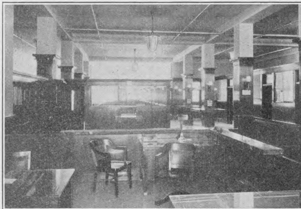
The above Bank has just been completed by us. Solid black Walnut Fixtures, with verdant marble trimming.
