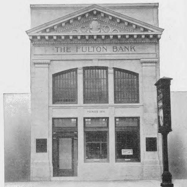
Fulton Bank, Fulton, Illinois Planned, Built and Equipped Under One Contract
