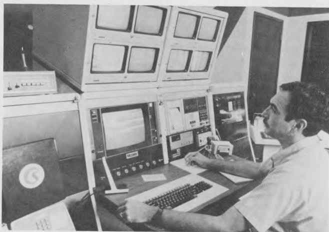
Mosler CCTV system monitors bank facilities, assets, customers and personnel.
