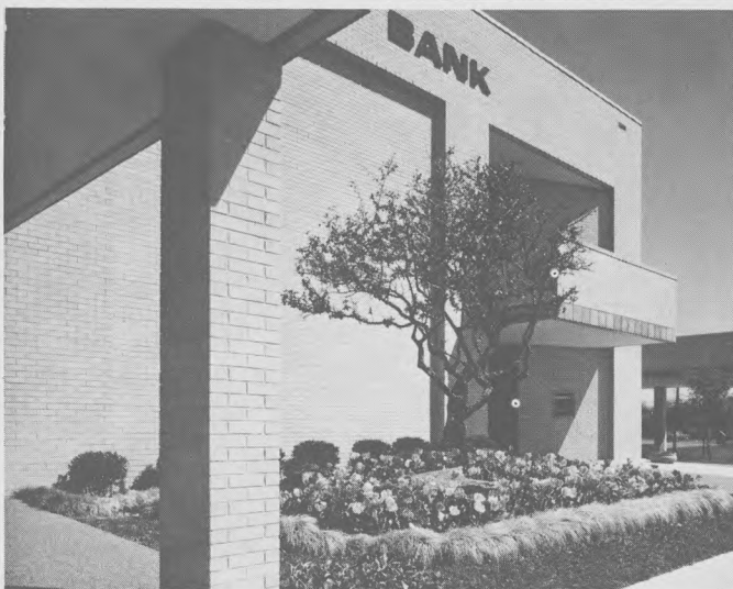
Commercial customers at new building for Guaranty Bank, Mt. Pleasant, Tex., have own entrance, shown at r. Entrance for retail customers is at l. Bank Building Corp., St. Louis, handled project.
