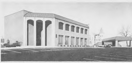
This is new Richmond branch of Wayne Bank, Cambridge City. Structure was erected as part of Richmond Redevelopment Plan.
