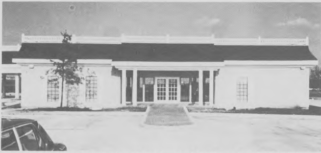
Exterior (above) and interior (below) of Willow Bend Nat'l, Plano, Tex. Exterior's high-roof chateau mansard with balustrade helps belie fact that structure is modular. Interior features period furnishings and oriental rugs. Son Corp., Wichita, Kan., supplied the building.
