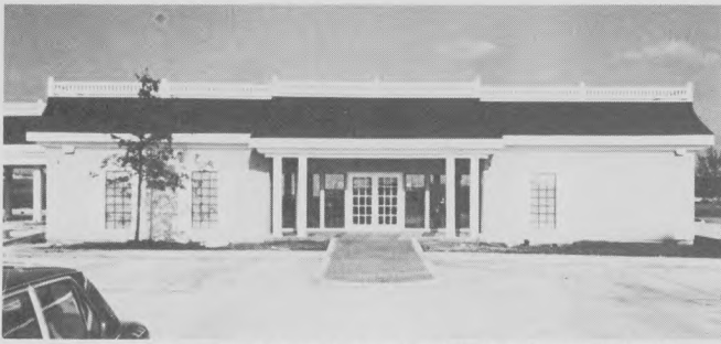
Exterior (above) and interior (below) of Willow Bend Nat'l, Plano, Tex. Exterior's high-roof chateau mansard with balustrade helps belie fact that structure is modular. Interior features period furnishings and oriental rugs. Son Corp., Wichita, Kan., supplied the building.
