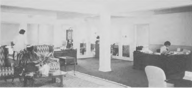
Two-story structure was built for Citizens Bank, Manhattan, Kan., to connect bank's original one-story building and a drive-up facility which had been 90 feet apart. Alvin Row, Architects, Lenexa, Kan., handled project.
