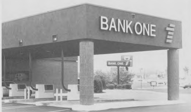
LEFT: Bank One's futuristic drive-up in Columbus, O., features overhead pneumatic-tube configuration that enabled bank to avoid costly installation of underground system in area with high water table. RIGHT: Troy (N.Y.) Savings Bank eliminated traffic
