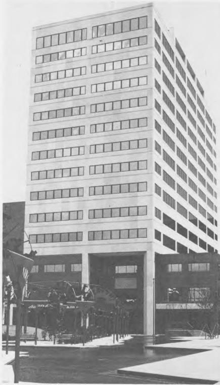
15-story Hancock Plaza is said to be tallest building between New Orleans and Mobile, Ala. Park-like area features pool, benches. 400-car garage adjoins building.
