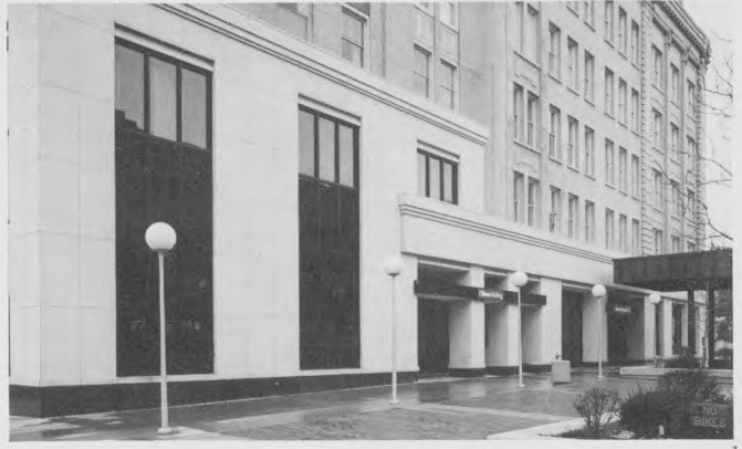
building. The two structures were tied together by a common front, as shown in these before (l.)-and-after (r.) photos. Bunce Corp., St. Louis, handled project.
