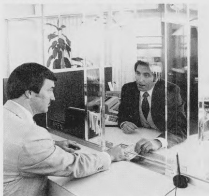
Bullet-resistant protective partitions from Mosler are manufactured of clear acrylic or polycarbonate.
