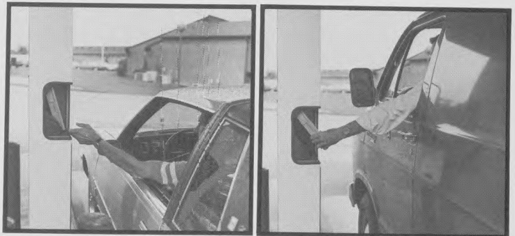
An AUTOVEYOR II carrier is easy to reach from a high or low driver's seat.
