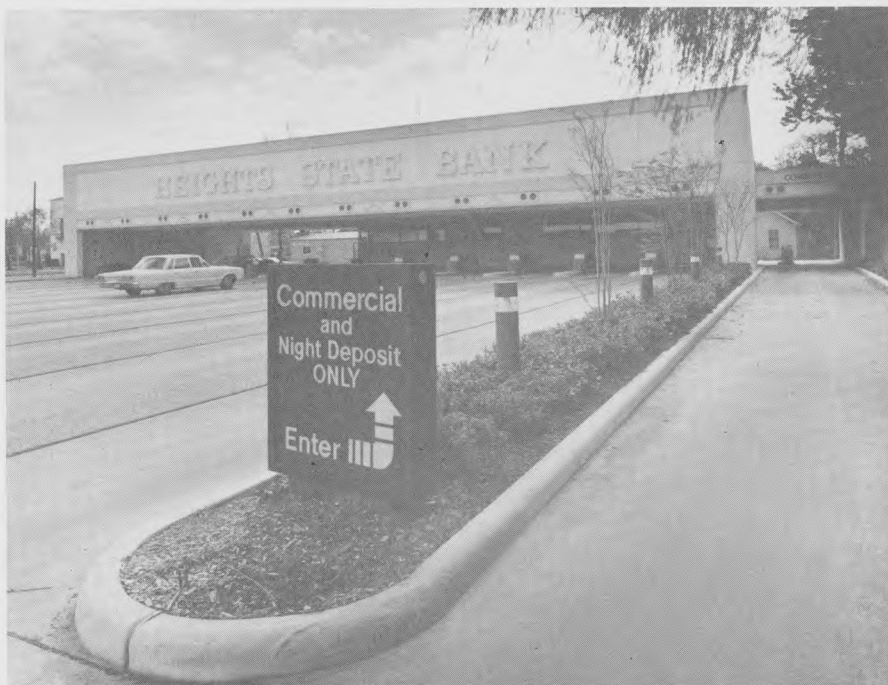
Retail and commercial traffic is segregated at Heights State, Houston, by signs and landscaped divider. Bank has 12 lanes for retail, two for commercial customers.
