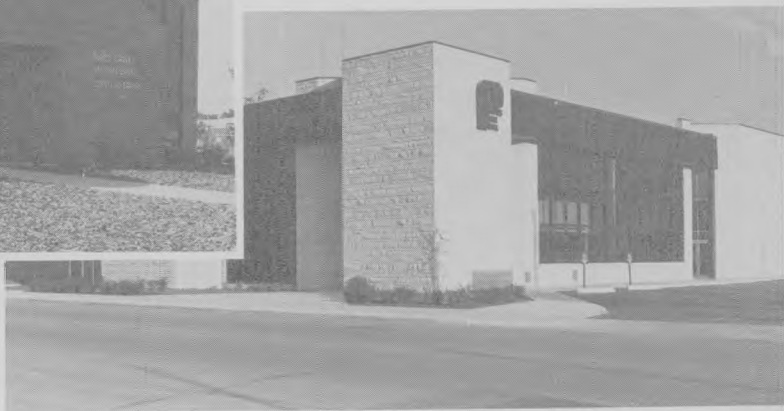
▲ Peoples State, Prairie Du Chien, Wis., a project of HBE Bank Facilities, St. Louis.
