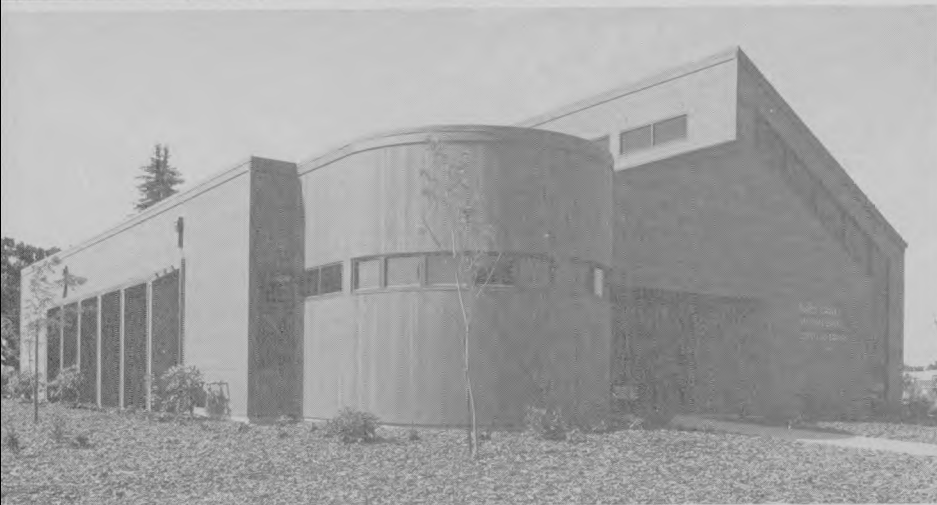
▲ Forest Grove National, Cornelius, Ore., a project of Bank Building Corp., St. Louis.
