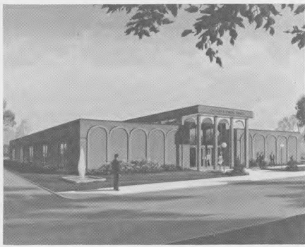
New building of Citizens State, Bald Knob, features contemporary design. Bank is observing its 50th anniversary this year.
