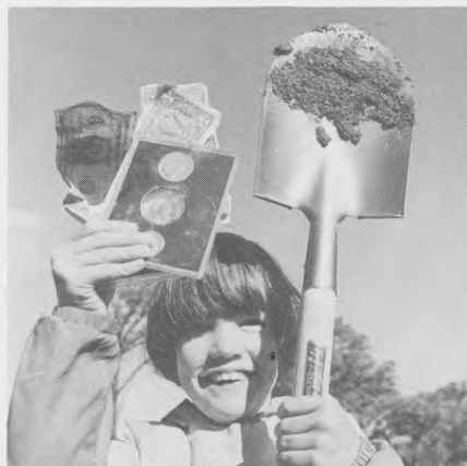
Eight-year-old proudly displays coins and currency she unearthed from construction site of Northbrook (Ill.) Trust during groundbreaking ceremonies featuring children enrolled at Horizon Children's Center. Funds were used by school to purchase equipment.
