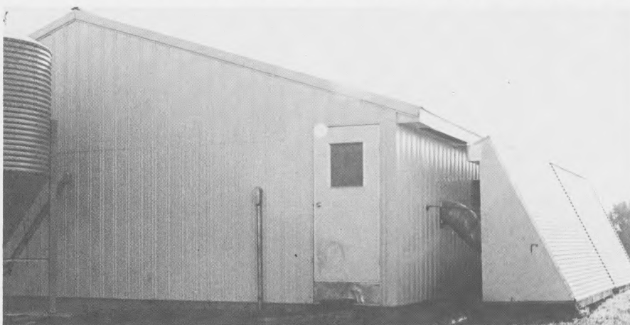
These two solar collectors (r.) are being used on Illinois farm to provide heat for building pictured. Because they are portable, they can be used to dry grain.
