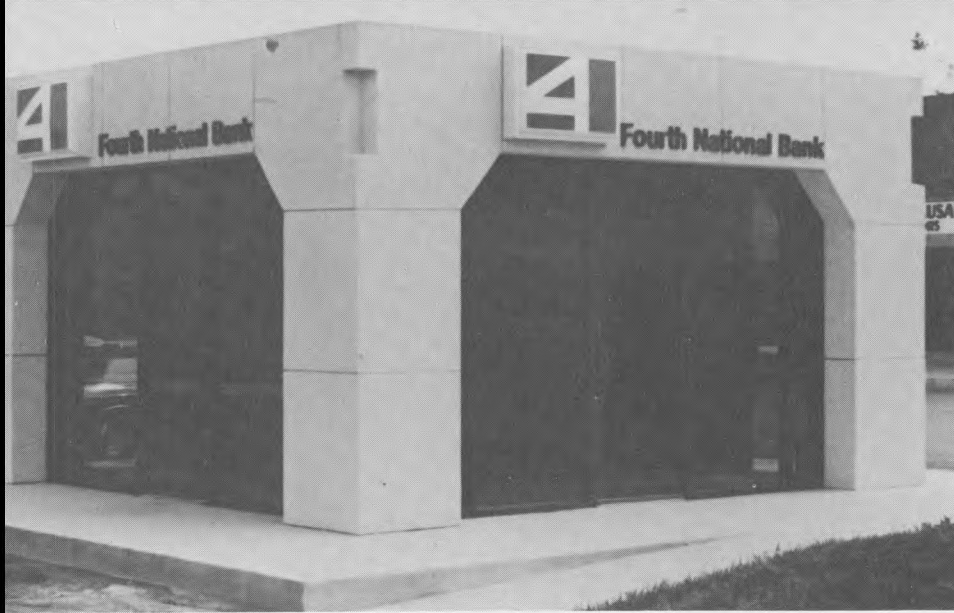
This free-standing building is example of structures Fourth of Tulsa erected to house its ATM network. They are located in shopping centers. Buildings were supplied by Cawthon Building Systems, DeSoto, Tex.
