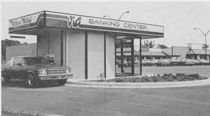
Customer uses drive-in ATM unit at Hutchinson (Kan.) Nat'l. Walk-in unit faces shopping center. Buildings are Diebold remote-transaction facilities.
