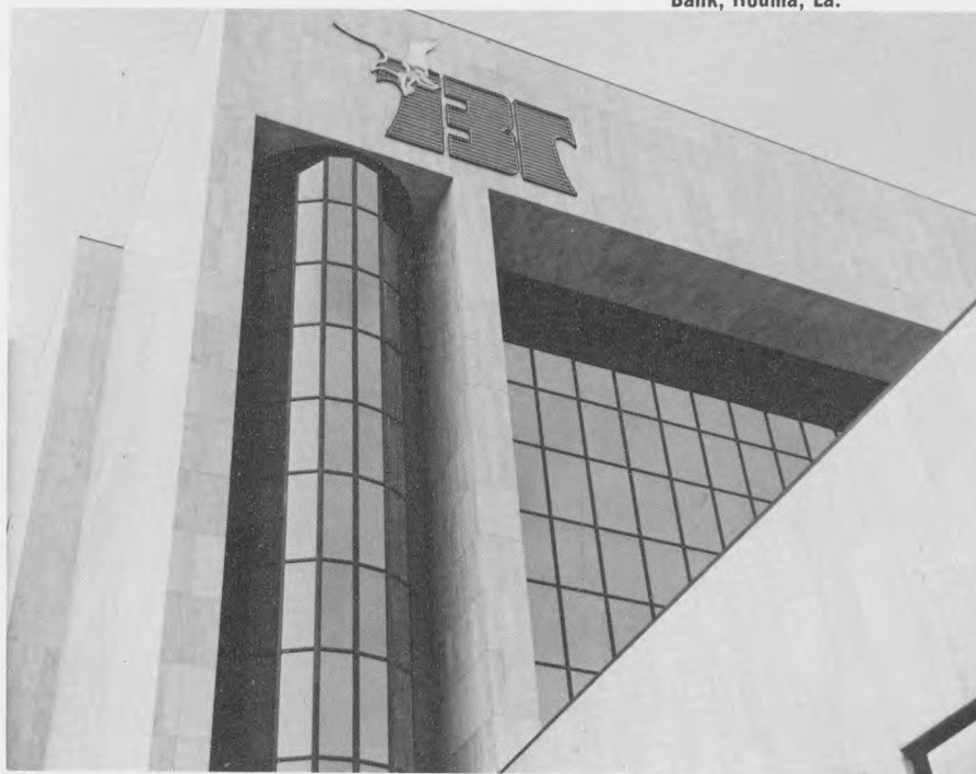
Contemporary 100,000-square-foot building features exterior materials of bronze setting integrated with white masonry panels.
