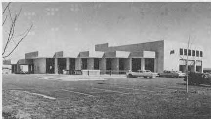
Garden National, Garden City, has opened new two-story building to replace former main bank. Old facility will be remodeled into detached office.
