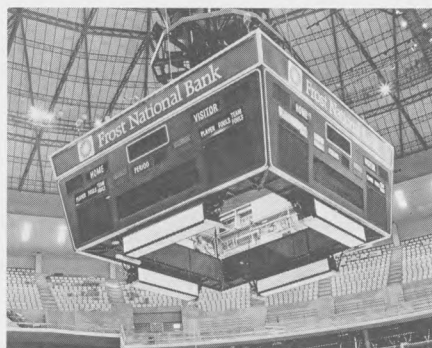
Frost Nat'l, San Antonio, purchased message center scoreboard for indoor sport use in city's arena. It is approximately 14x28 feet, weighs 10,000 pounds, contains more than 12 miles of wiring and has 12,504 lamps that can spell out messages.
