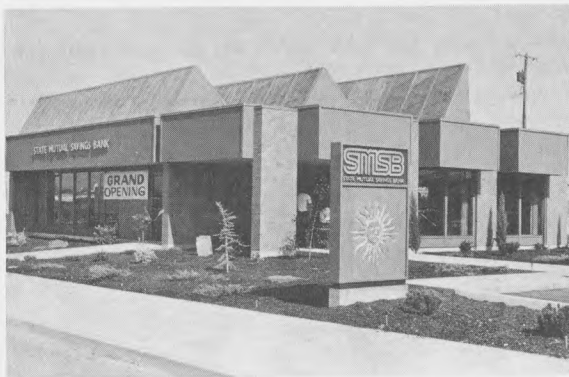
TOP: Home Savings' solar branch features special architecture to blend in with Norwegian heritage of Stoughton, Wis., where it's located. Solar panels on steep roof collect energy to heat bank and provide hot water. BOTTOM: Three peaks of solar collectors accent roofline of State Mutual Savings office in Othello, Wash., which is said to be first solar-heated financial building in state.
