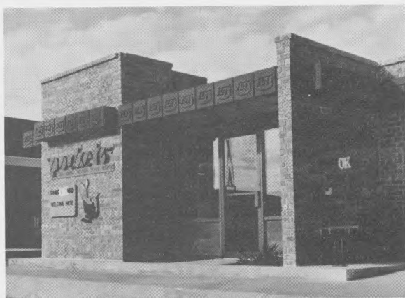
One of six "Pockets" ATM facilities operated by First Nat'l, Stillwater, Okla. During introduction of units, transactions were authorized via orbiting satellite.
