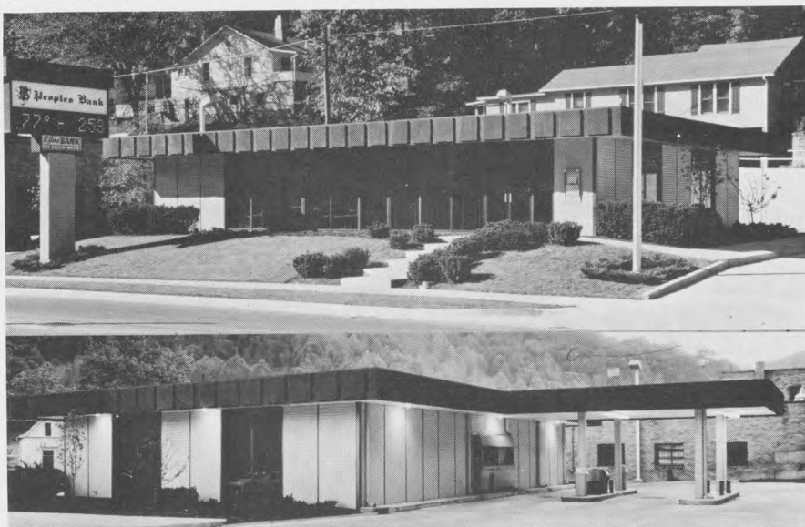
TOP: Front view of pre-manufactured building housing Peoples Bank, Hazard, Ky. BOTTOM: Side view of bank shows drive-up at rear of building. Structure was made by Diebold Financial Buildings, Clearwater, Fla.
