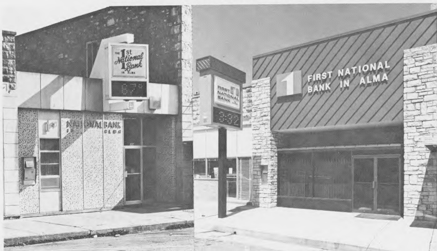
These photos show the dramatic effect a facelift can have on a bank building! At l. is facade of First Nat'l, Alma, Kan., prior to remodeling by HBE Bank Facilities Corp., St. Louis. At r. is finished job, which features native fieldstone pilasters and solar bronze colored glass in windows and doors.
