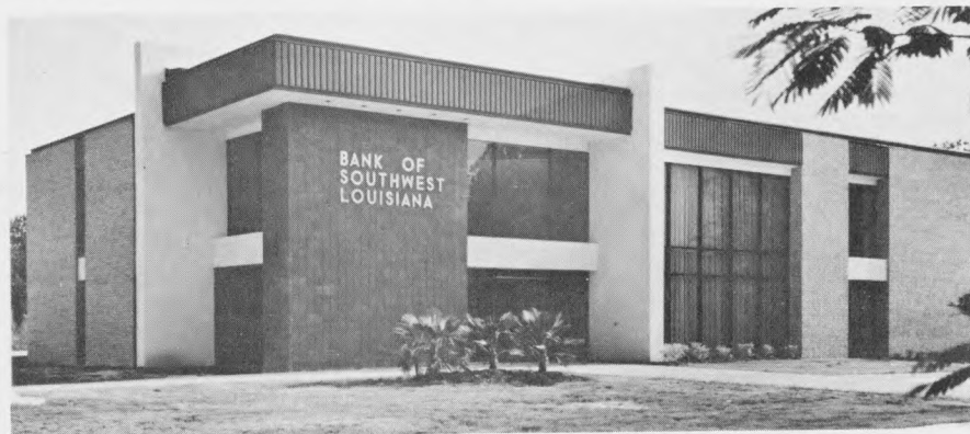
This new home of Bank of Southwest Louisiana, Oakdale, is example of pre-engineered building.
