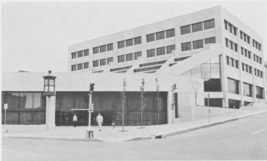
New quarters for American Nat'l, St. Joseph, Mo., and Ameribanc, Inc. (foreground) are part of Robidoux Center, which stands on site formerly occupied by Hotel Robidoux. Artifacts from hotel and old bank are featured in bank. One of them, old Empire Trust Co. clock, hangs near main entrance.
