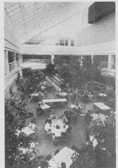
Continental Bank covered light court (bottom) of original building with tubular steel and glass skylight to create two-story atrium (right), which contains employee cafeteria and lounge areas. New floor of atrium covers original roof. Trees and plants heighten outdoor effect.
