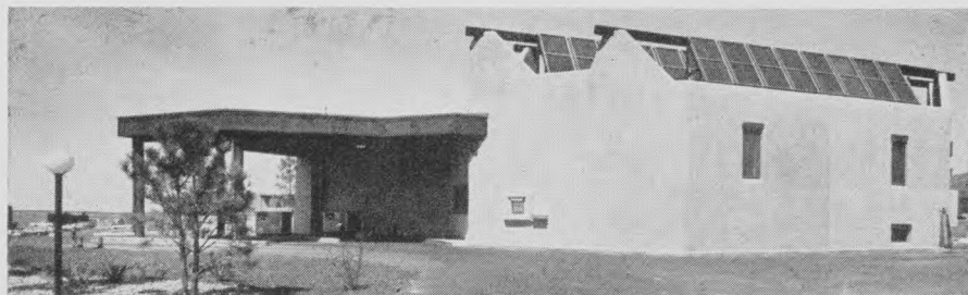
Rooftop solar panels can be seen best from rear of new facility of United Southwest Nat'l, Santa Fe, N. M. This is said to be first facility in nation to rely on solar energy for basic heating, cooling needs.
