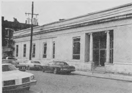
Main Office of First State, Pineville, Ky., was being remodeled before flood hit last April.
