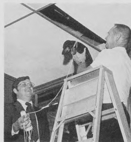
"Puppy power" comes to rescue at Merchants Nat'l, Mobile, as Gene Harkey (r.), property and purchasing engineer, and Russell Harris, v.p. and br. mgr., place Mr. Harkey's dog, Friskey, in area above ceiling to run wiring for automatic teller. Space above false ceiling was too small to admit human, so Friskey was called on to assist.
