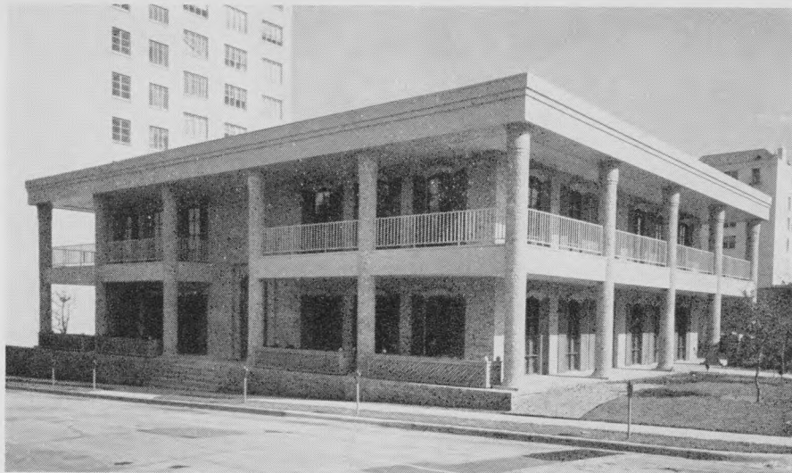
New headquarters building of Texas Bankers Assn. in downtown Austin is located directly across street from governor's mansion. Designed in Texas colonial style, $1.2-million structure is TBA's first home of its own in its 92-year history.
