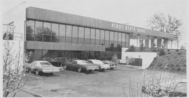
Wide expanse of temperate insulated solar bronze glass windows on lower level contrasts with exposed aggregate precast panels on building's top level.
