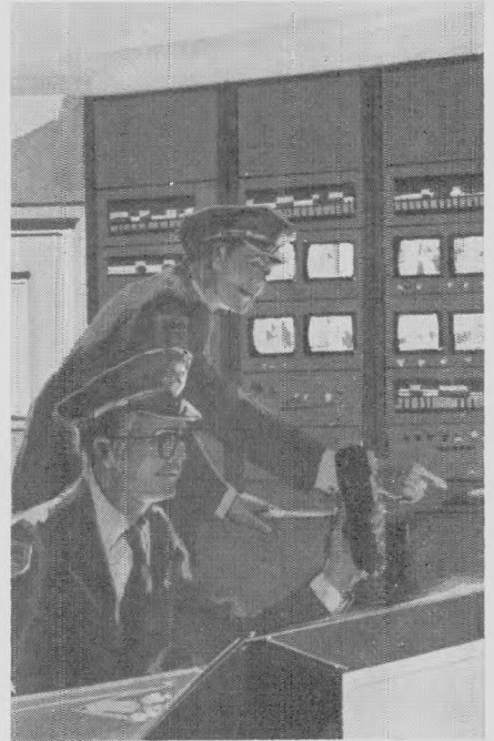
Mosler proprietary alarm system located in sub-level of bank enables security officers to monitor entire building.
