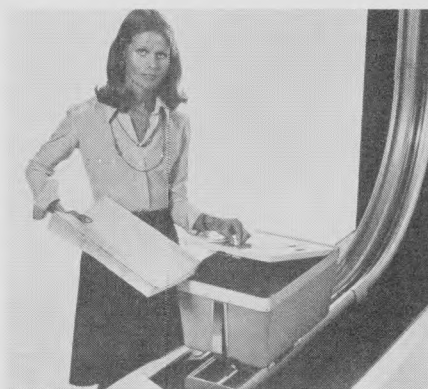
Bank personnel can place up to 20 pounds of paperwork in each Telelift car and send car on its way to other departments via automated delivery system supplied by Mosler.
