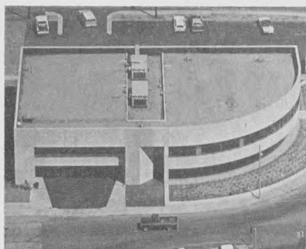
This aerial view of new quarters of First Nat'l, Wynne, shows unusual curved design of building's front. Structure is designed with mezzanine that encircles lobby.
