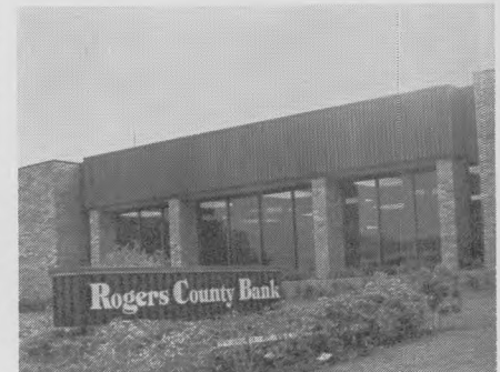
Brick parapet walls ranging in color from buff to dark beige dominate the exterior design of Rogers County Bank, Claremore, Okla. A bronze-finished metal fascia and full-length solar bronze windows accent the building's front; the bank's drive-up was refurbished to complement the design. Rogers County Bank's canopied drive-through protects customers entering the lobby in bad weather. Inside, terra cotta and burnt orange dominate and a fireplace is the center of attraction in the oak-paneled waiting area. Also decorating the open-space interior are several original paintings, including a valuable oil of Will Rogers.
