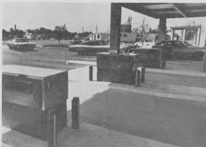
West Xenia Branch's new facility includes this six lane, inline drive-up using Diebold equipment. Drive-up reportedly is longest in state.
