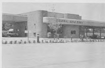
Above are front and rear views of drive-up facility of Central Bank, Farmers Branch, Tex. Accompanying article tells how bank "redid" its motor bank so that it serves more customers than old facility did, but with little increase in personnel.
