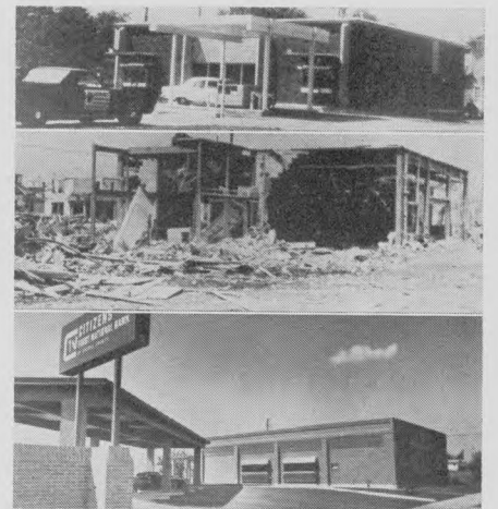
TOP: West Xenia (O.) Branch of Citizens First Nat'l, Xenia, before tornado of April, 1974, struck. CENTER: After tornado, only portion of foundation, vault remained in usable condition. BOTTOM: 13 months after storm, new building was opened. Is larger than original, boasts features that set precedents for area.
