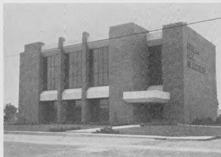
The new Main Office of Citizens Bank, Hartselle, Ala., is three stories tall and has drive-up facilities in a separate building on its lot. The Main Office design is massive brick vertical columns that surround the window areas. Offsetting the verticals are horizontal lines of aggregate concrete that shade the first- and third-floor windows from suniight.
