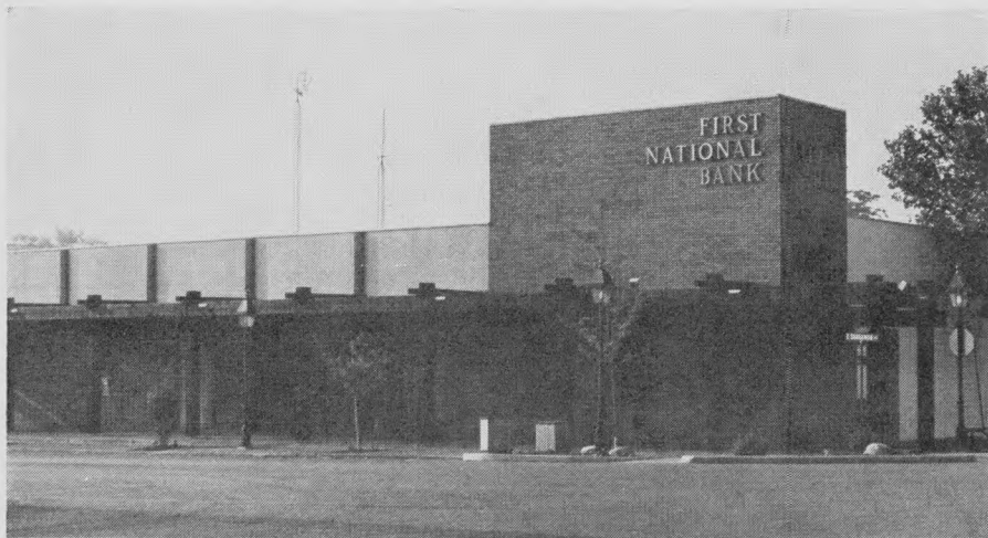
This building formerly housed dime store, but was converted into new quarters of First Nat'l, Rantoul, Ill. Structure is across street from bank's old location. Plate-glass storefront gave way to red brick. Large cedar posts support canopy along front and part of side of building.
