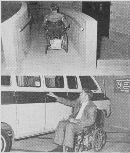
TOP: Ramps from Mercantile Bank of St. Louis' parking garage to its tower and Eighth Street building provide easy access for handicapped.
