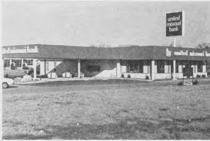
This is United Missouri of Springfield's new facility's quarters. Building formerly housed hamburger stand, but was completely redesigned, obliterating all traces of past use.
