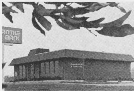
This is the new home of Mercantile Bank of St. Charles County, St. Charles. Bank Building Corp., St. Louis, was the consultant and construction manager for the project.
