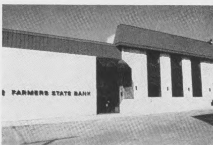
Newly remodeled and expanded quarters of Farmers State, Cameron, feature new entrance covered by glass canopy. Glass walls have been added and entire interior has been redone. Grand opening featured punch and cookies made by banker's wives. Contest for guessing number of coins in a jar offered savings accounts of $100, $75, $50 and $25 as prizes.
