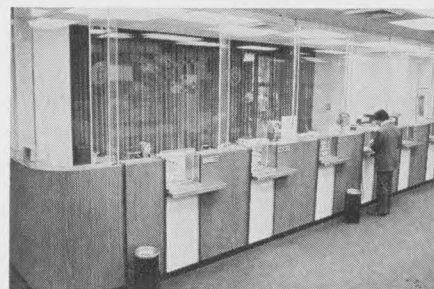
Enclosures of DuPont "Lucite" provide security and open appearance, as can be seen in this lobby photo of First Federal Savings of Philadelphia's Downtown Branch. Manufactured and marketed by the Wilmington, Del., company, transparent plastic is abrasion and bullet resistant.
