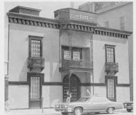
Look of old New Orleans was captured on remodeled exterior of Madison (Ind.) Bank building. Wrought iron balcony and railings are complemented by unique molded-glass windows and circle-headed and beveled-glass entrance.
