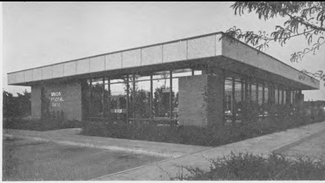
LEFT: Union Nat'l, Wichita, opened facility in this pre-engineered building supplied by Butler Manufacturing Co. Structure was erected under design/build system, which, according to Butler, shortens building timetable considerably. RIGHT: Interior of Union Nat'l facility features integrated lighting/ceiling panels, part of Butler's Space Grid system.
