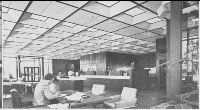
LEFT: Union Nat'l, Wichita, opened facility in this pre-engineered building supplied by Butler Manufacturing Co. Structure was erected under design/build system, which, according to Butler, shortens building timetable considerably. RIGHT: Interior of Union Nat'l facility features integrated lighting/ceiling panels, part of Butler's Space Grid system.
