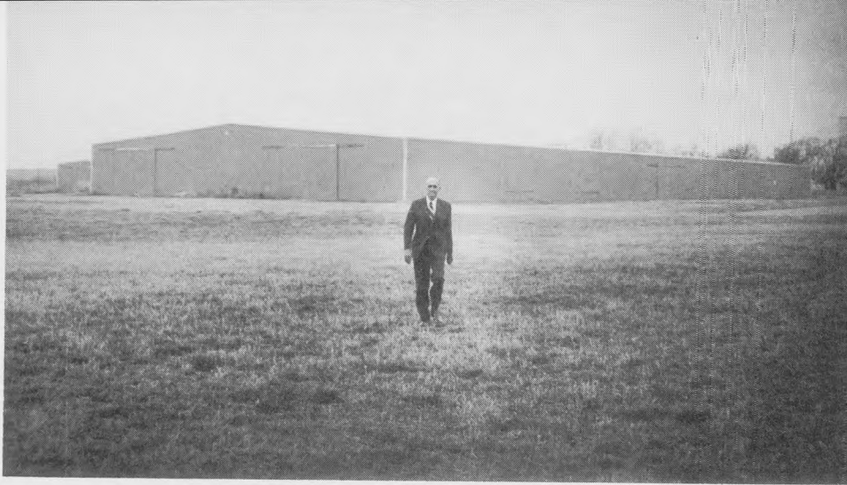
Mr. Duwe, always active in his community, was in large part responsible for bringing this 62,000-square-foot manufacturing company to Lucas. The firm makes double-wide mobile homes and has provided about 50 jobs. Mr. Duwe helped negotiate purchase of the site and arranged the financing to attract the industry to Lucas.
