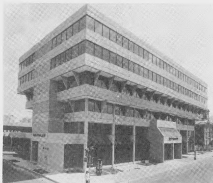
This is new home of Bank of Springfield, featuring cantilevered design that gives building appearance of inverted pyramid.
