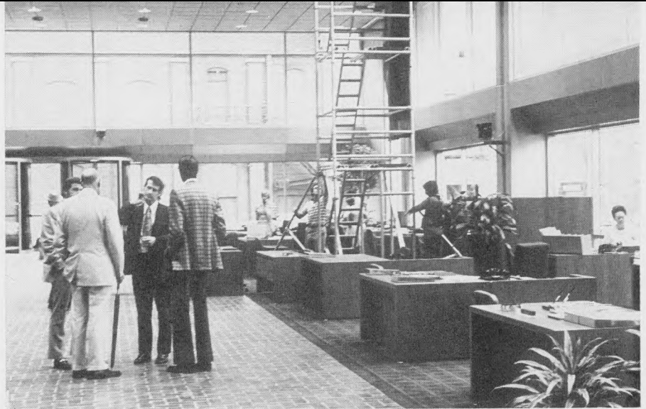
Bank representatives chat with customers in new two-story lobby while workmen complete ceiling, which is coffered, faced with chrome.
