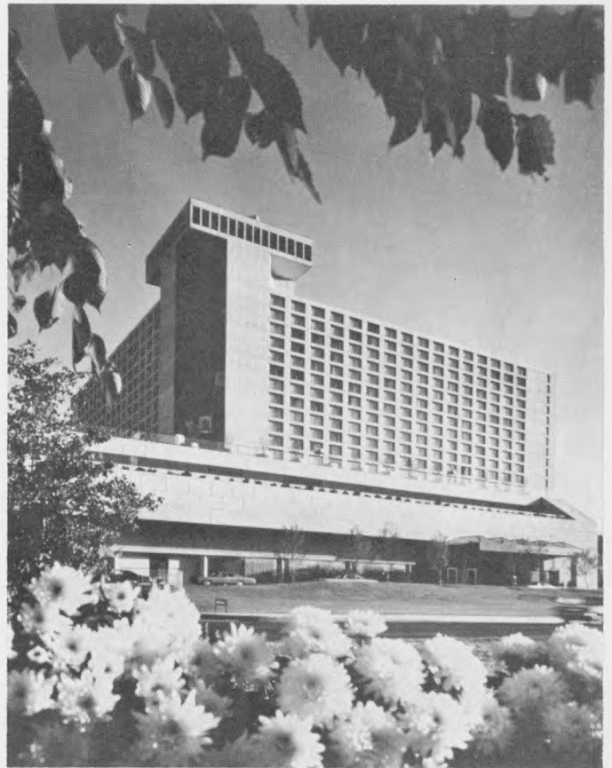
15 story hotel is perched atop 70 foot high limestone bluff. Five-story function block at base of bluff contains convention facilities. Penthouse dining area at top of hotel is served by glass-enclosed elevators.
