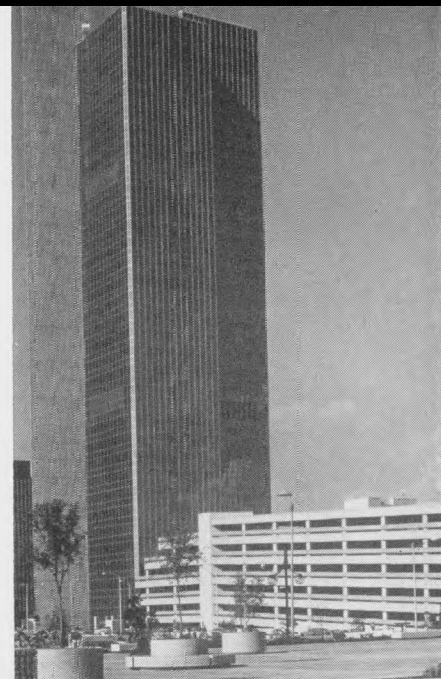
Shown here are Valley Bank Center and eight-story parking garage in Phoenix, subject of recent joint ownership purchase agreement between Valley Nat'l, Phoenix, and Prudential Insurance.
