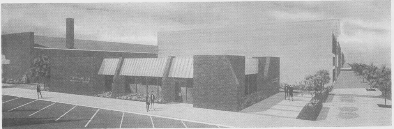
Exterior of Chandler National's new building will be brick with bronze anodized settings and bronze glass. Stained wood fascia panels (with downlighting) will be situated over landscaped areas. Planters will face the town square.
