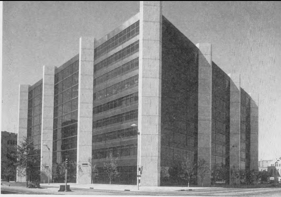
Fourth Financial Center building, home of Fourth of Wichita, is clad in bronze-tinted glass with concrete pylon supports.
