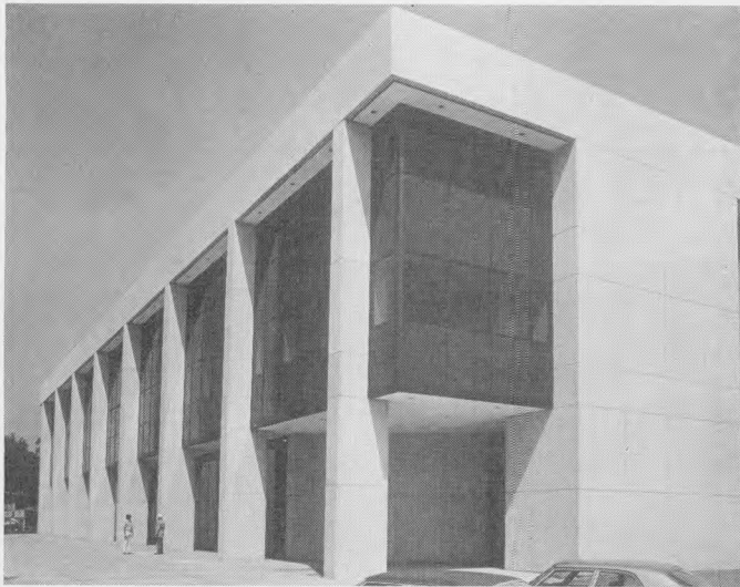
Exterior of Bossier Bank is of structural steel, clad in warmtone concrete of sandblasted limestone aggregate with bronze-tinted glass.
