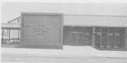
This is First-Cannelton National's new home, which was dedicated June 2. Drive-up facilities are shown at left.
