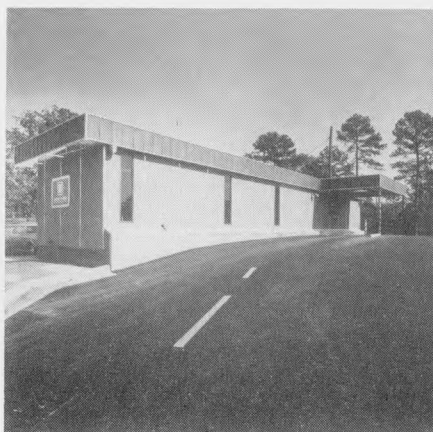
Rear of Worthen facility shows drive-up window and driveway. After-hours depository is located under canopy.
